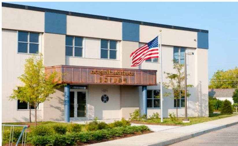
South Burlington Police Department
