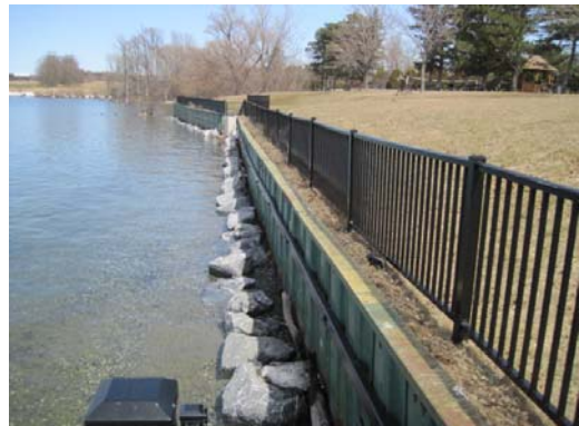
Shelburne Town Beach Wall
